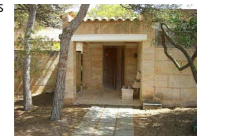
71 Jørn Utzon: architect's house, Porto Petro, entry porch
