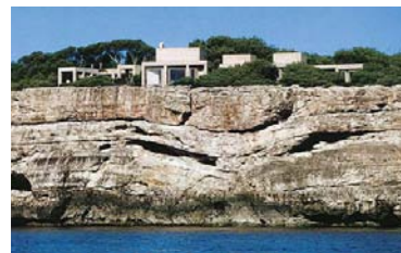
52 Jørn Utzon: architect's house, Porto Petro, Majorca, Spain (1972)
