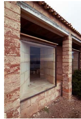
72 Jørn Utzon: architect's house, Porto Petro, 'eye socket' windows
